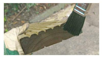
Timber which is rip sawn, equalised, planed or heavily sanded must be returned to the treatment plant for retreatment.
