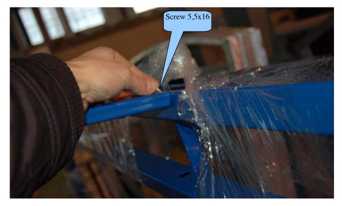
6.Fix the roof tapes on two middle roof beams (Nr. 8 on General Arrangement Drawing) using screw 5,5x16.
