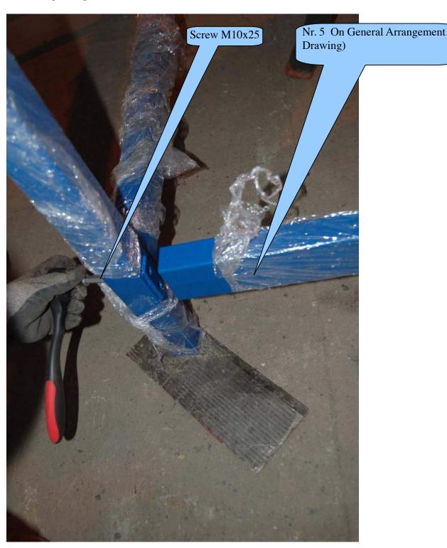
4. Fix the middle posts (Nr. 6 on General Arrangement Drawing) as with screws M10x25
