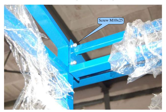
3. Fix the steel construction of FRONT WALL (Nr. 5 on General Arrangement Drawing) with side wall (Nr. 1 on General Arrangement Drawing) and with the front wall post (Nr. 7 on General Arrangement Drawing) using screw M10x25
